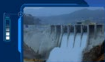
HUA NA HYDROPOWER PLANT
