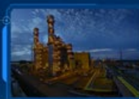
CA MAU 1 - 2 THERMAL POWER PLANTS
