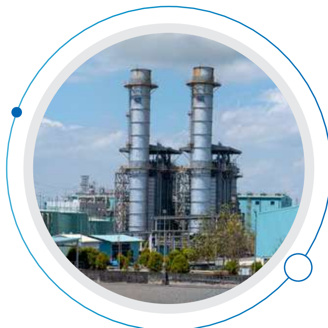
PETROVIETNAM NHON TRACH POWER COMPANY NHON TRACH THERMAL POWER PLANT 1
