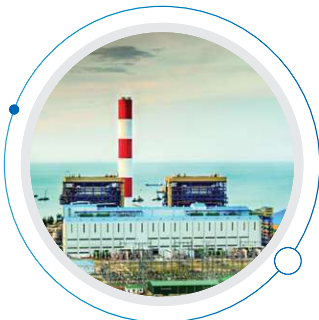
PETROVIETNAM HA TINH POWER COMPANY VUNG ANG 1 THERMAL POWER PLANT
